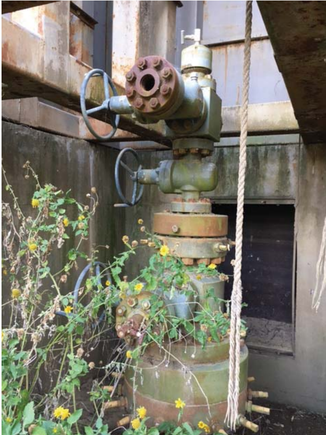
Primero-1 Well, drilled in 2006, with a flow rate of 2.8 mmcf/d (Cattle Creek Formation) reported from this well
